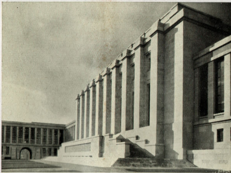
Main Façade of Assembly Building
